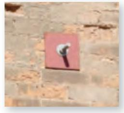
A steel plate with anchor bolts.
