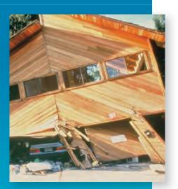
The walls around the garage door of this home were not strong enough to withstand the shaking of the 1989 Loma Prieta Earthquake.
